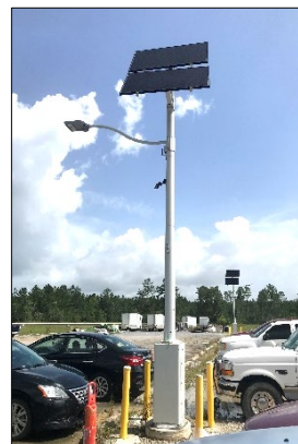
Photovoltaic and LED light poles in parking lots. Pictured here are B-4124 and B-8000 parking lots.
