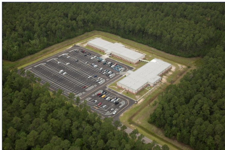
Buildings 3225 and 3226 are on their way to earning LEED certification.
