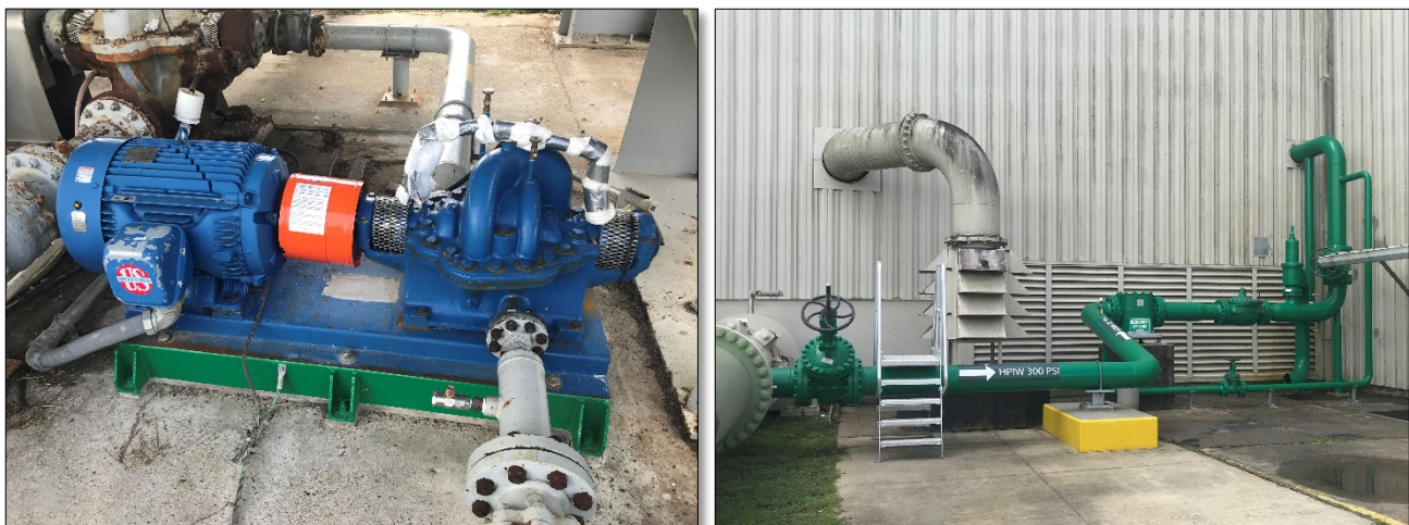
B4400 UESC Implementation: Installation of a high-efficiency pump and motor assembly.
