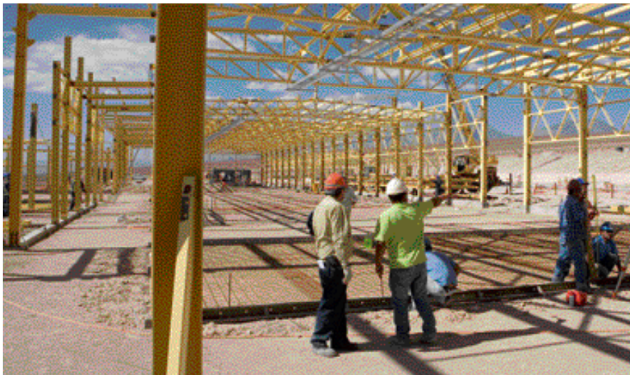
Construction of the OSF Technical Buildings.
