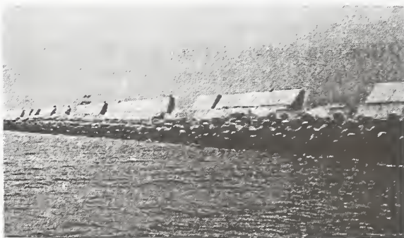
Photo 4 Seawall in the artificial island off the Shin-Moji Port
