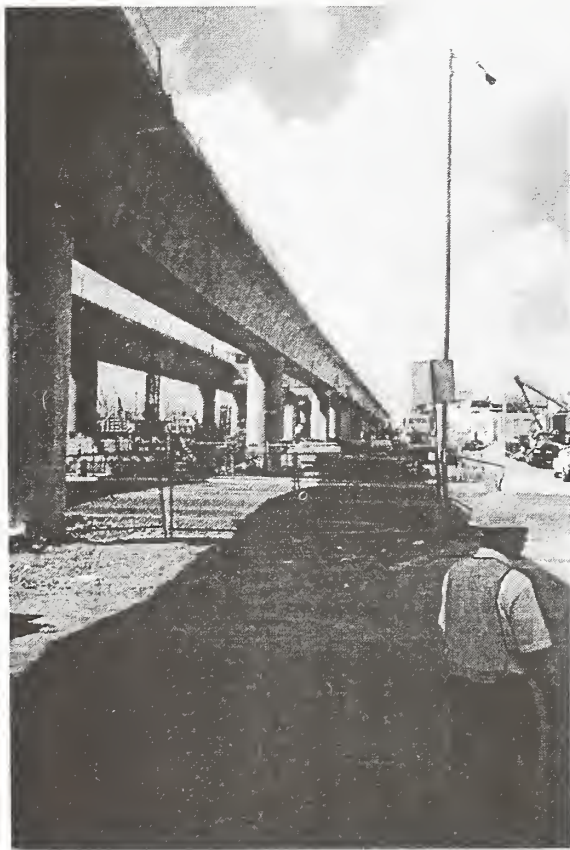
Figure 6: Elevated guideways under construction in Bayamón.
