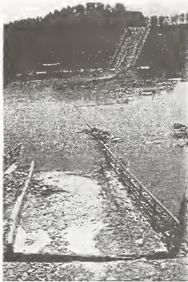
Photo 8 Collapse of Sakarya Central Bridge
