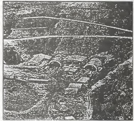
Figure 26: Bolu Tunnel at Asarsuyu Portal
