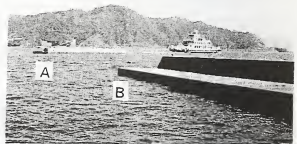
Photo 3 Breakwater in Odo Port
