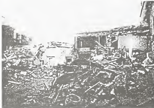
Photo 21 Damage of sundried brick structure (Tungshih, Taichung County) It is completely destroyed. It is near the building of photo 7.
