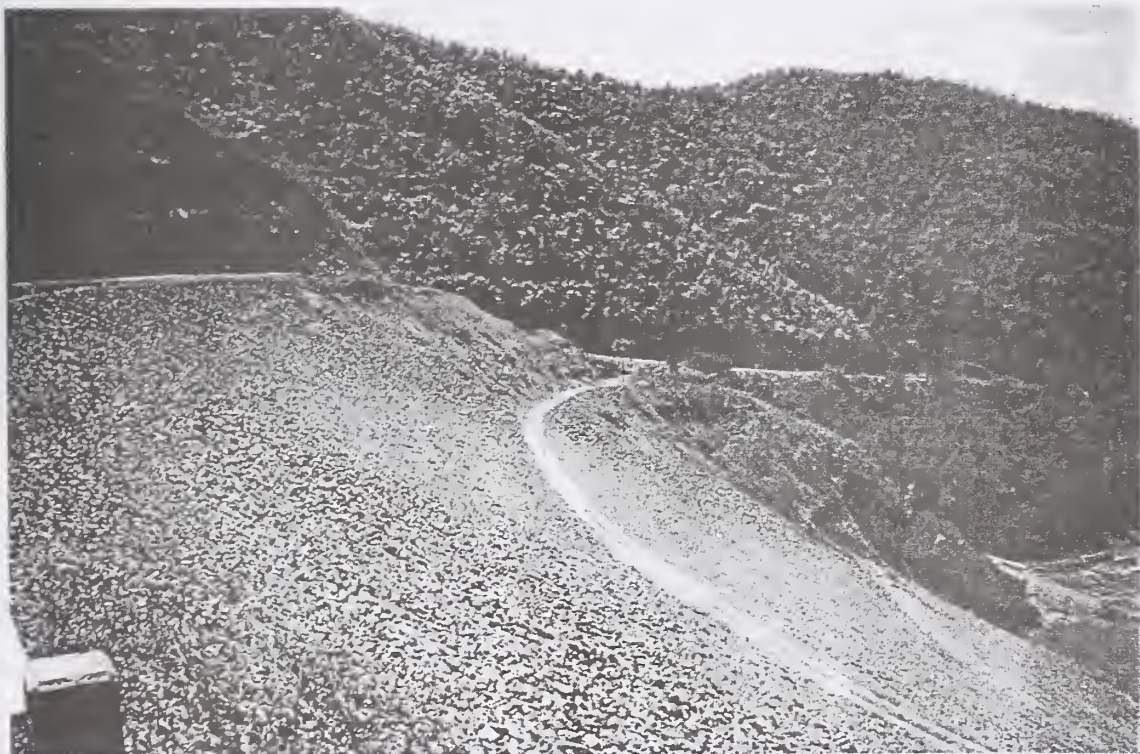
Figure 3: View of Cerrillos Dam embankment.
