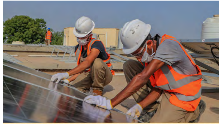
Workers install solar panels to power a public hospital in Yemen, restoring operations affected by ongoing conflict.
