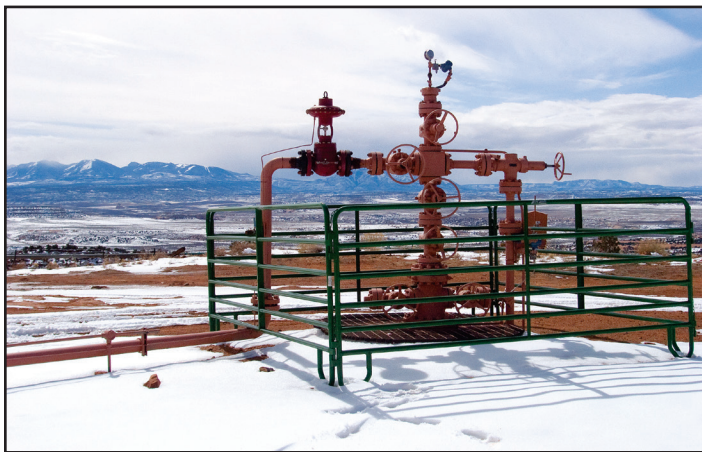
Natural gas wellhead at the Lisbon field, southeast Utah
