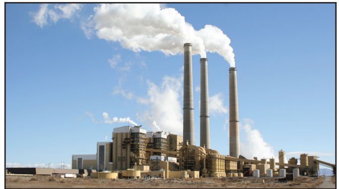
Hunter coal-fired power plant
