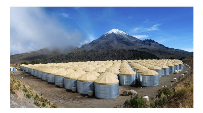
The HAWC Observatory, perched next to a volcano at an altitude of 13,500 feet, uses its 300 massive water tanks to scoop up the products of high-energy particle collisions happening in the upper atmosphere. Credit: Jordan Goodman
