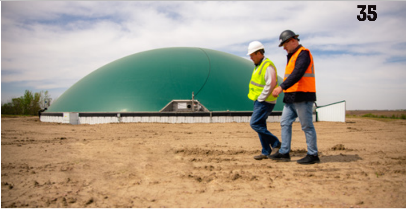
Right: Bob Powell at the Athena project site where anaerobic digesters convert methane from cow waste into renewable natural gas and fertilizer. Below: Powell walks in front of bales of plastic to be recycled at Brightmark's circularity center in Ashley, Indiana.
