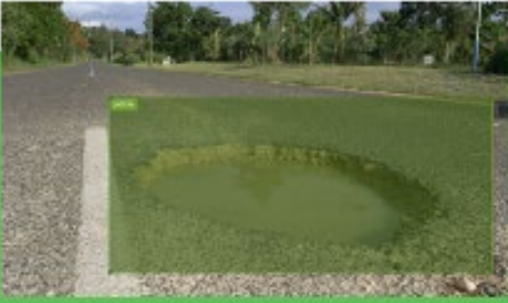
Identification & Detection of potholes through machine mounted camera module and using Computer Vision & AI
