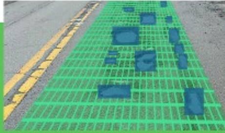
Calculating the area of potholes repaired by using LIDAR. Complete transparency in terms of the material used and work done
