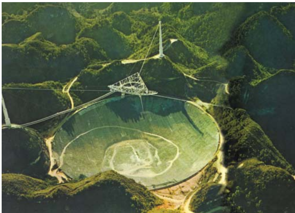
Fig: 11.17: The Radio Telescope near Arecibo, Puerto Rico : One of the biggest and most sensitive of its kind, this radio telescope located in a natural bowl in a mountain has a 300 m wide dish of wire netting. Radio waves emanating from the sky are reflected by the dish to an overhead aerial that is moved for focussing on different astronomical objects.
