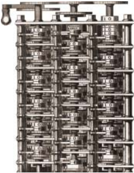
Fig: 19.6: The Difference Engine of Babbage automatically produced mathematical tables.
