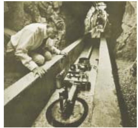
Fig: 15.3: 72 feet quartz rod strain seismograph in a mountain tunnel.
