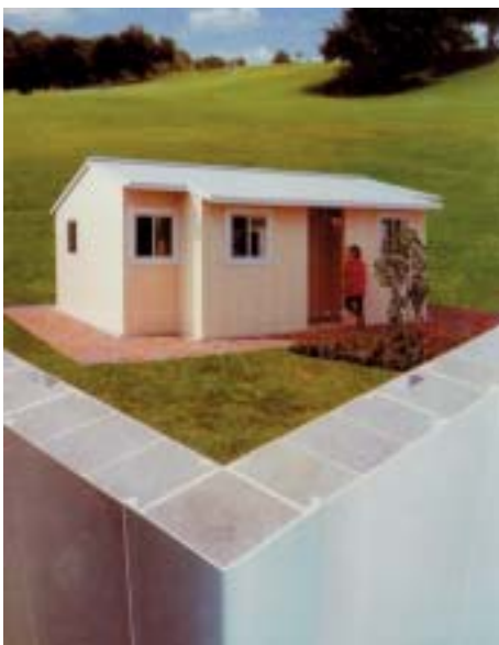
Fig: 17.41: House of Plastics: The walls, floors, roof and everything within are made of synthetic plastics. Even lawns and pavements are available in plastics.
