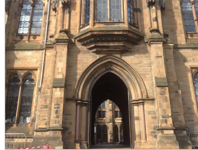
Main Building 253 and 250 Main Entrance, G12 8QQ
