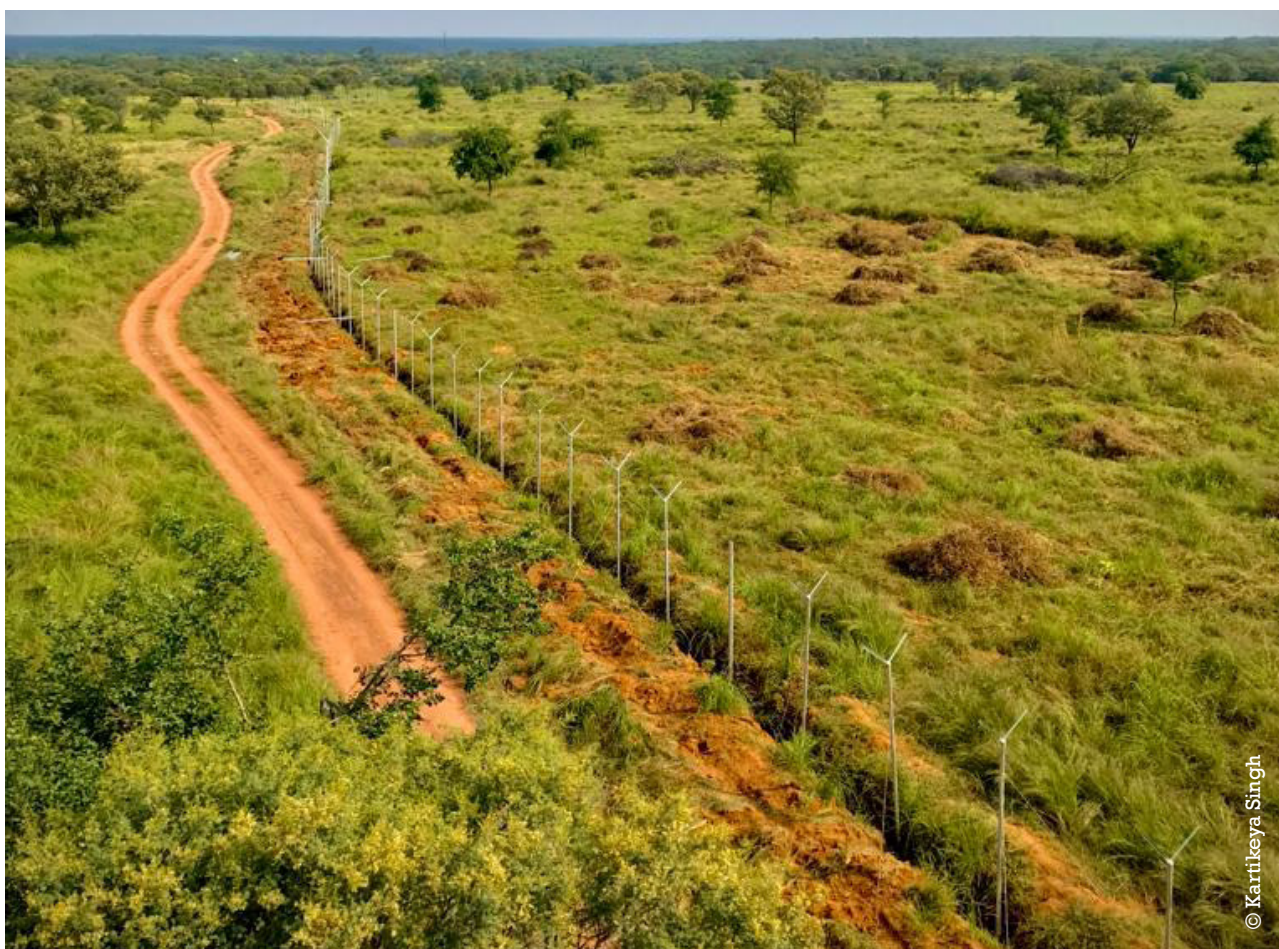
Image 7. Predator proof fenced enclosure under construction for soft release of cheetahs in Kuno National Park.
